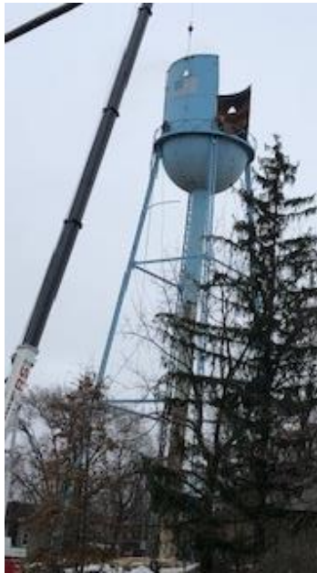
Demolition of the old Smithfield Water Tank took place in December of 2019
