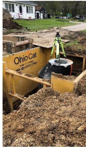
GPS Surveying equipment is used to ensure accurate locations and elevations of all pipes and manholes
