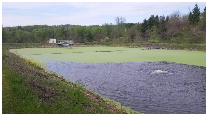
One of the two aerated lagoons located at the Smithfield Wastewater Treatment Plant. These lagoons create an aerobic environment which promotes the natural breakdown of wastewater solids.
