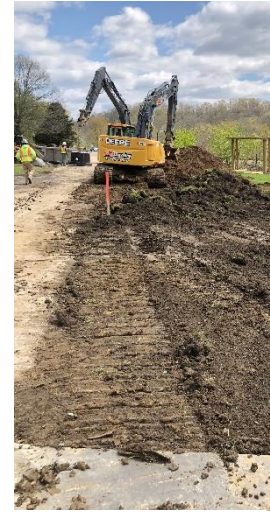
Excavators digging out and backfilling trenches for pipeline installation
