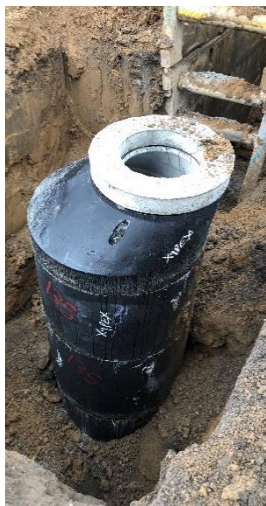
A newly placed sanitary manhole
