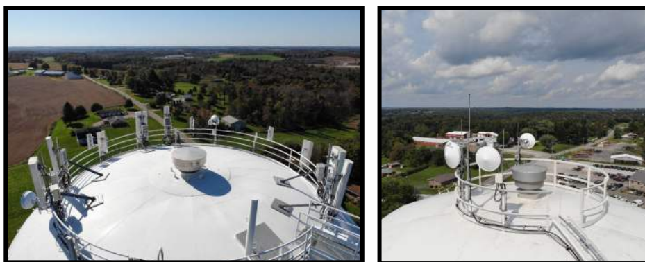
The JCWSD Regularly Inspects all of their Water Storage Facilities, and pays special attention to the equipment mounted on top of the various elevated tanks throughout the county. Equipment mounted on top of these tanks includes the JCWSD's SCADA and Telemetry System Antennas, as well as cellular and radio antennas for local communication companies and service providers. Two photos from the 2022 inspection flights of the very top of two elevated water storage towers, with heights of 100ft and 130ft, are shown above (2022).
