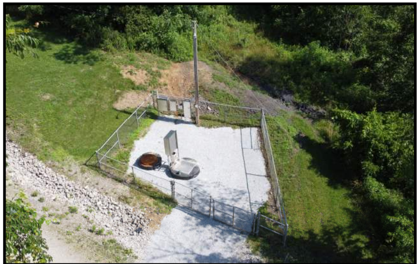
One of the nine pump station sites that has been rehabilitated as part of this project. The pump station construction included the installation of two brand new pumps, new pump control panels, valve vaults, and effluent force mains (2023).
