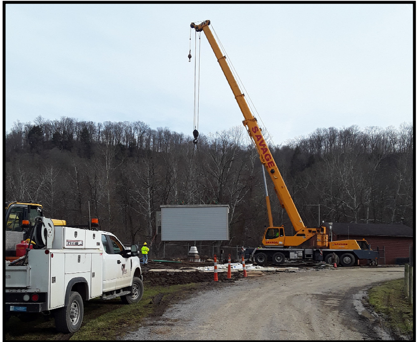
The new prefabricated electrical building was lifted into place via crane onto the site (2022)
