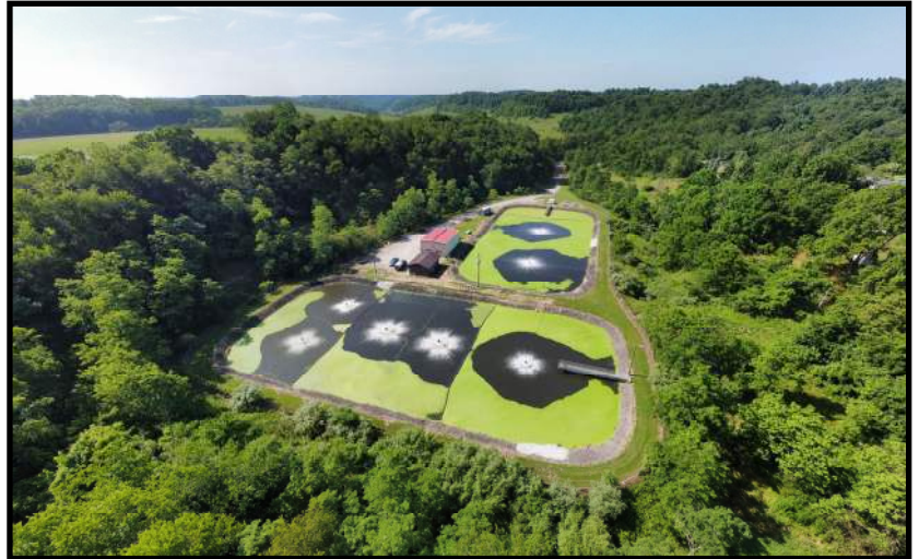
The dual Lagoon setup at the Smithfield WWTP, post rehabilitation in the summer of 2023. The upgraded WWTP includes floating aerators, baffling, dredged lagoons, and a UV disinfection tank (2023).
