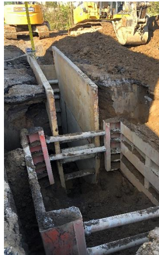
Trench boxes are used to protect workers against cave ins while laying pipes and setting manholes
