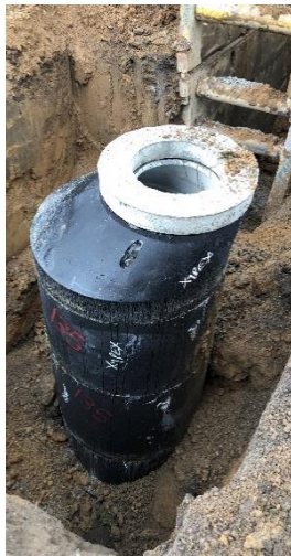
A newly placed sanitary manhole
